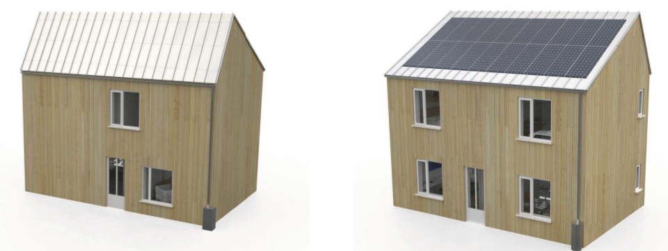
The core house is shown at the end of Phase 1a, clad throughout in vertical timber boarding, with a standing seam aluminium roof.
