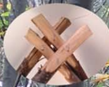
Photo of 1:10 scale model showing jointing at ridge
