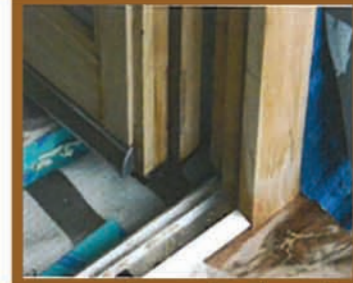
joinery, insulation and weatherproofing
