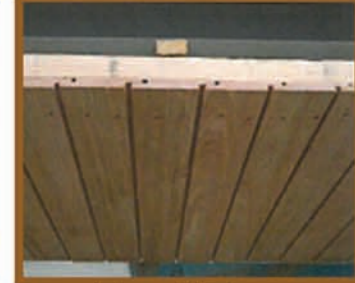
external / internal finishes & services
