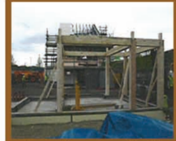
foundations, delivery & assembly of frame
