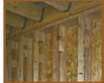
infill panel components & pod installed
